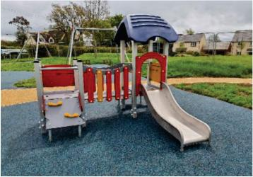
**Finding:** The item has been installed marginally too high which has resulted in the platform height being in excess of 600mm (630mm) and technically, the height of the barriers (550mm) are now insufficient to meet the requirements of BS EN 1176 Part 1. This is however a very low risk technicality and no remedial action is recommended as it has not affected the risk assessment of the item
