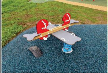
**Finding:** The grass surface forms part of the impact area around the equipment and the surface has not yet established
