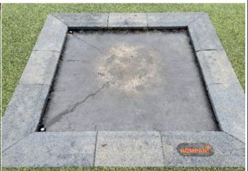
**Finding:** On site visits it is not possible to test the ground clearance of the Bouncing Facility bed as specified in BS EN 1176; ensure that the clearance between the Bouncing Facility Bed and the ground underneath is in accordance with the manufacturers recommendations
