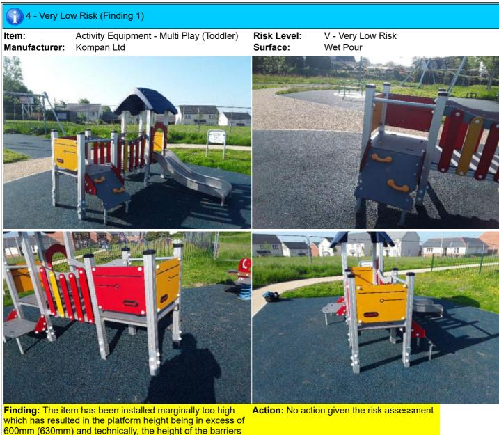
which has resulted in the platform height being in excess of 600mm (630mm) and technically, the height of the barriers (550mm) are now insufficient to meet the requirements of BS EN 1176 Part 1. This is however a very low risk technicality and no remedial action is recommended as it has not affected the risk assessment of the item
